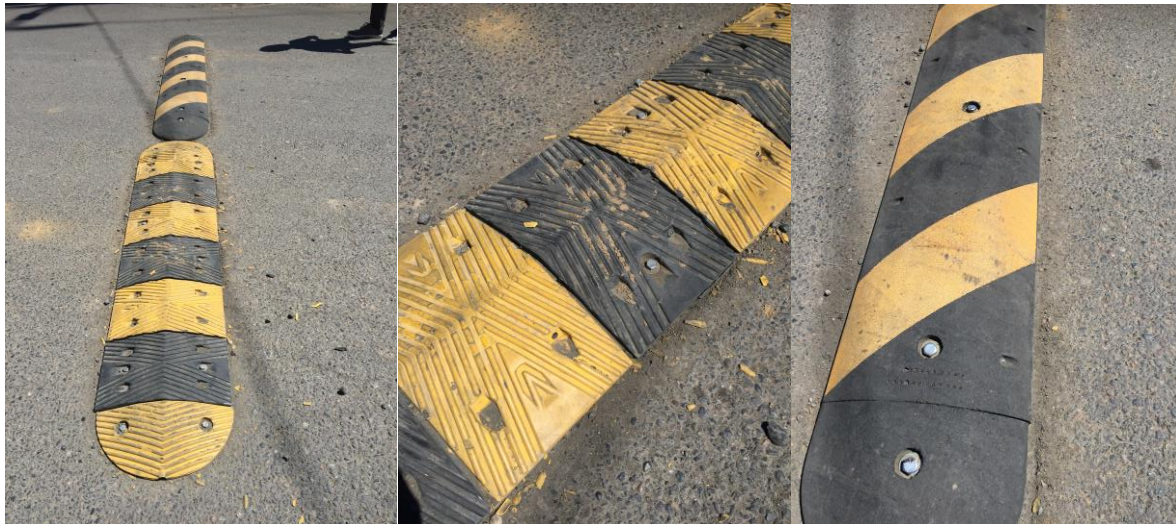
The TreeTop Products bump (left photo at front and middle photo) and Checkers bump installed for testing at a PBOT parking lot, pictured after approximately two months of use.
