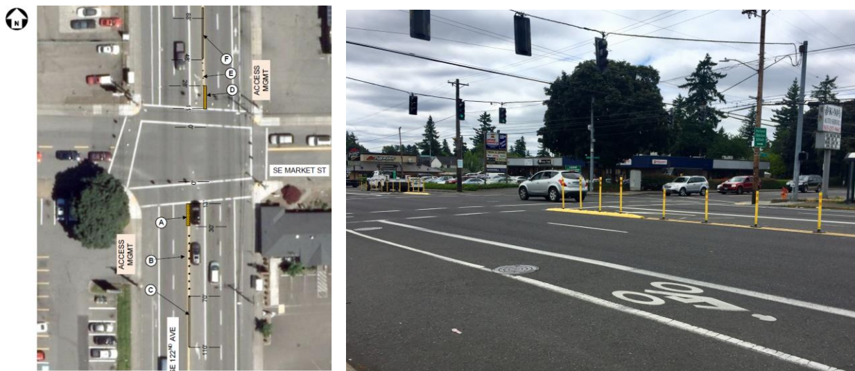
Figure 7. A PBOT work order (left) shows a top-down view of a hardened centerline using plastic curbing and delineators (labeled "A") that is extended to support access management (B) on the south leg of SE 122 nd Ave. & Market St. The photo (right) shows the installation looking north/northeast.
