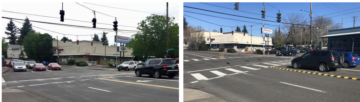
Figure 11. PBOT installed high-visibility crosswalks concurrent with left turn calming, including at SE Holgate & Chávez boulevards, pictured on May 20, 2019 (left) and on March 9, 2020, afterward.
